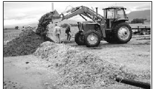
The formation of an aerated windrow. Note the straw that is placed over the pipe to increase porosity.
